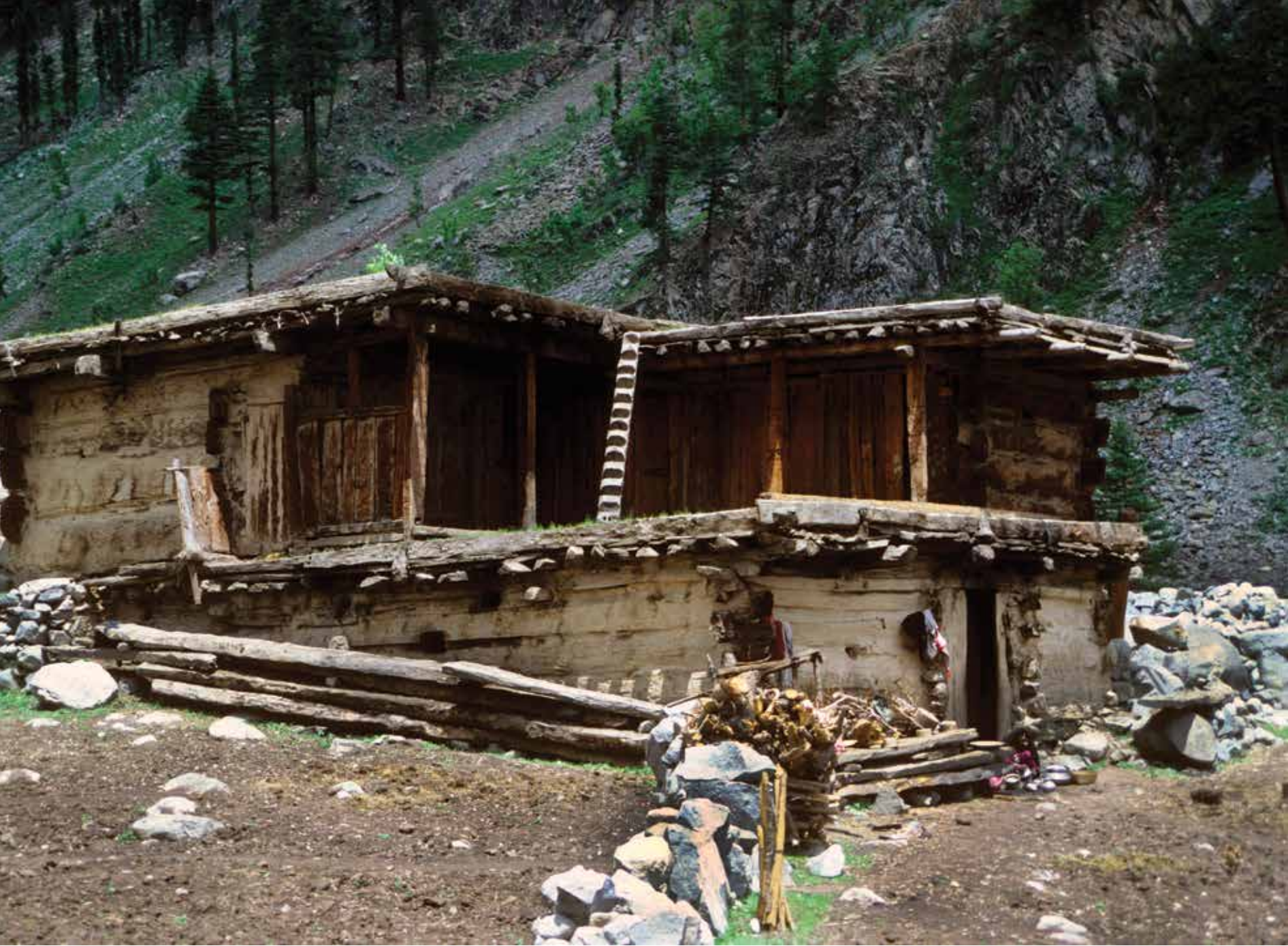
A two-storey farmhouse in Bara Jabba built from assembled tree-trunks. 1983.
