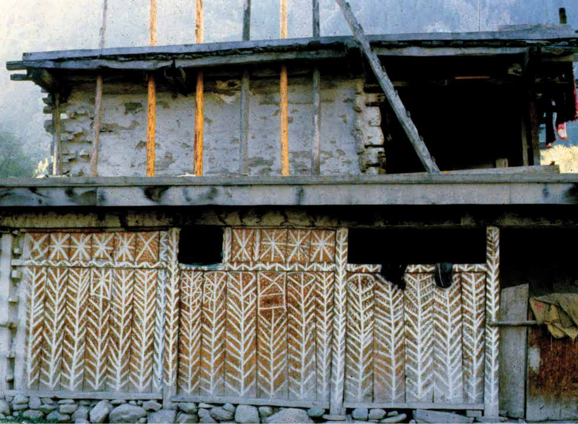
A two-storey farmhouse in Kalam Kas with standing wooden poles to store hay. The wooden wall framework with white tree-like patterns is built to keep privacy of the household. 1985.
