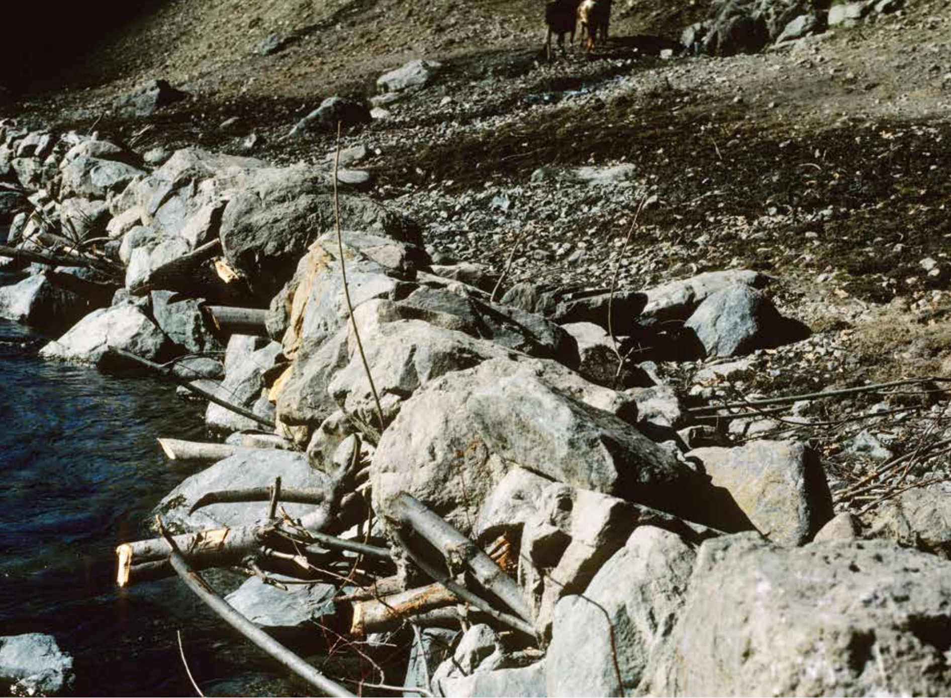
A protection wall made of stone and tree branches built by local people to protect newly cultivated field from the river. 1983.
