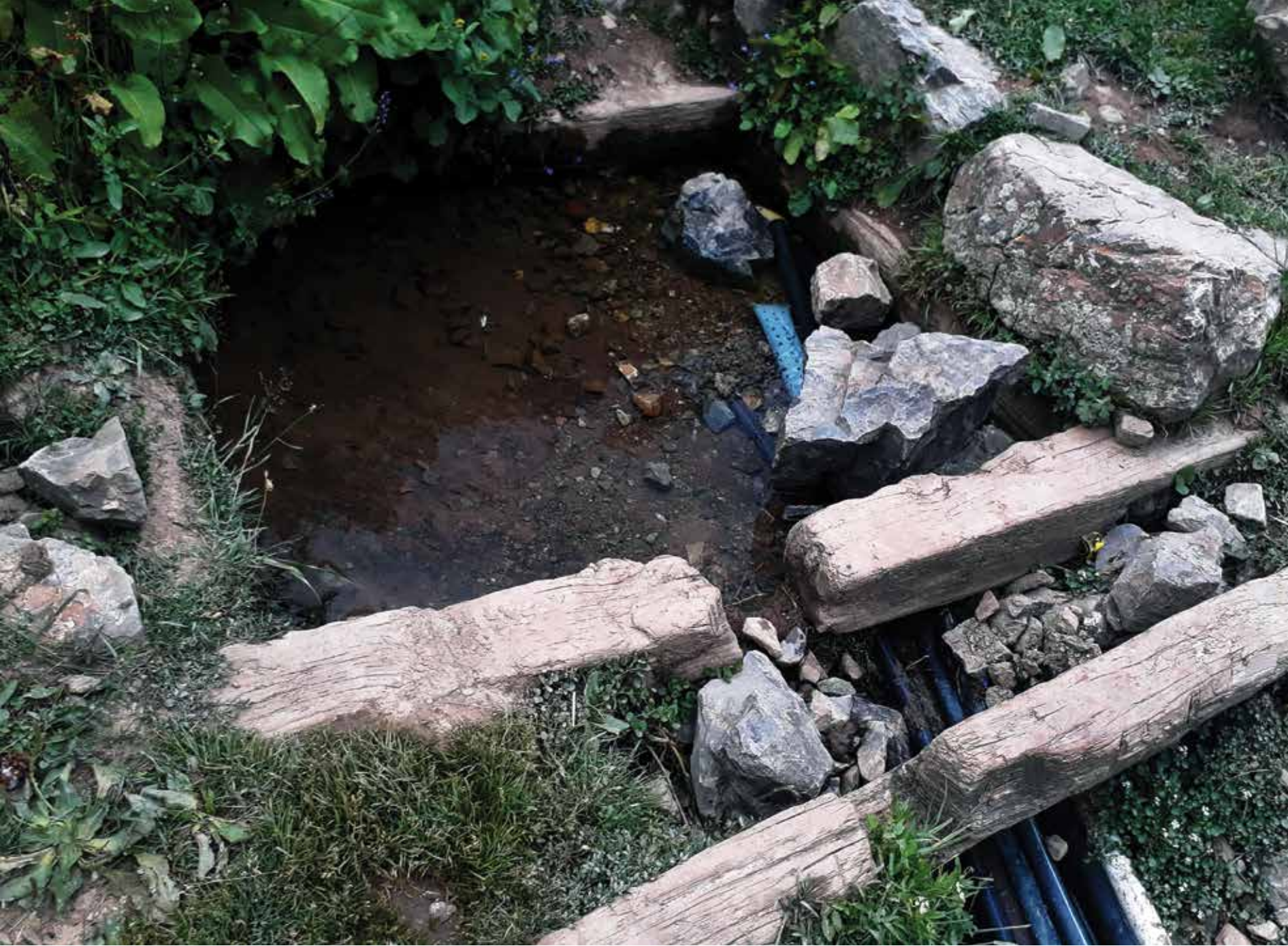
Tap drinking water with plastic pipes from a natural source near mosque at Boyun. 2019.
