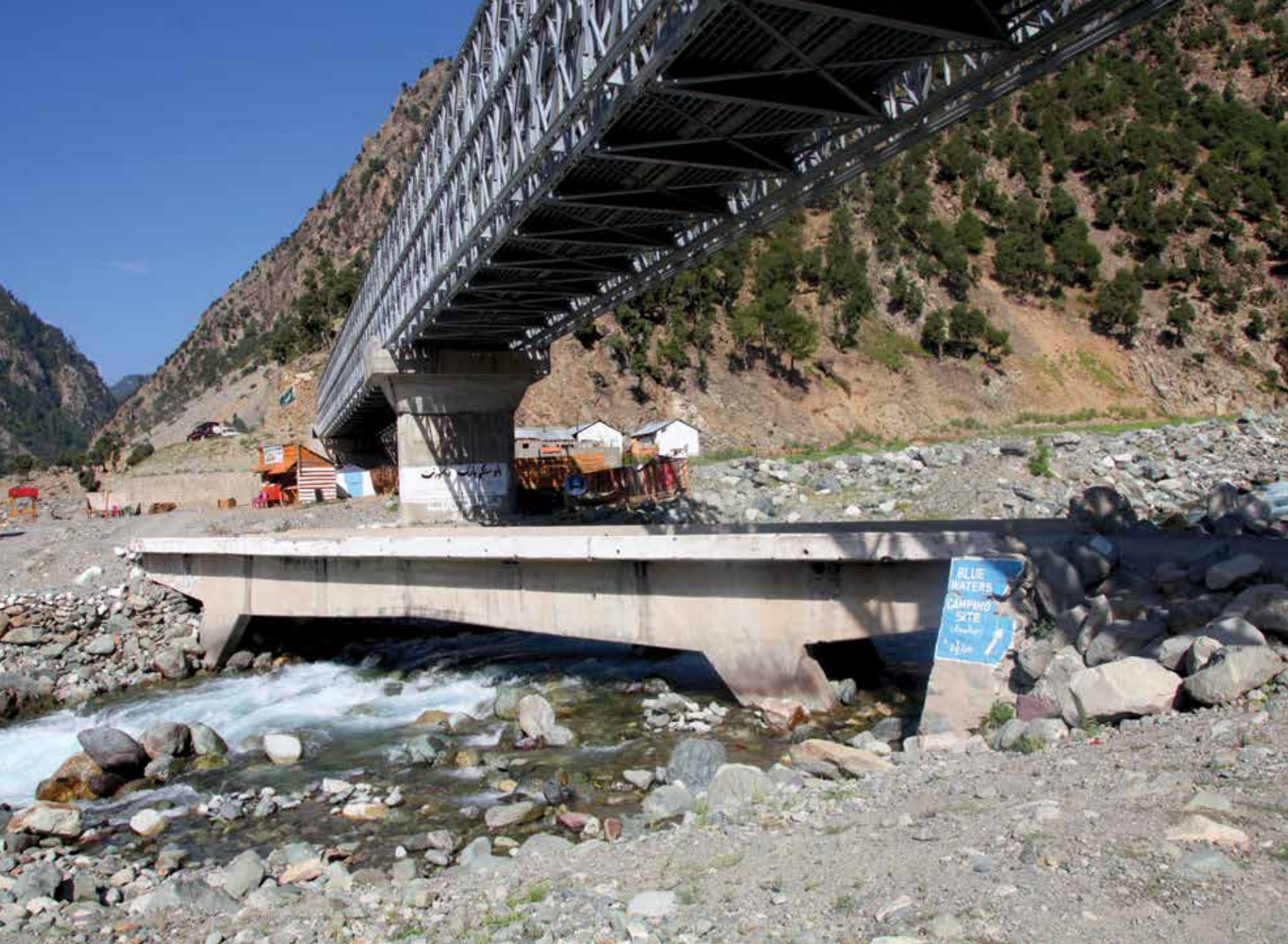
The old and new bridge in Bhan over Anakar River. 2019.
