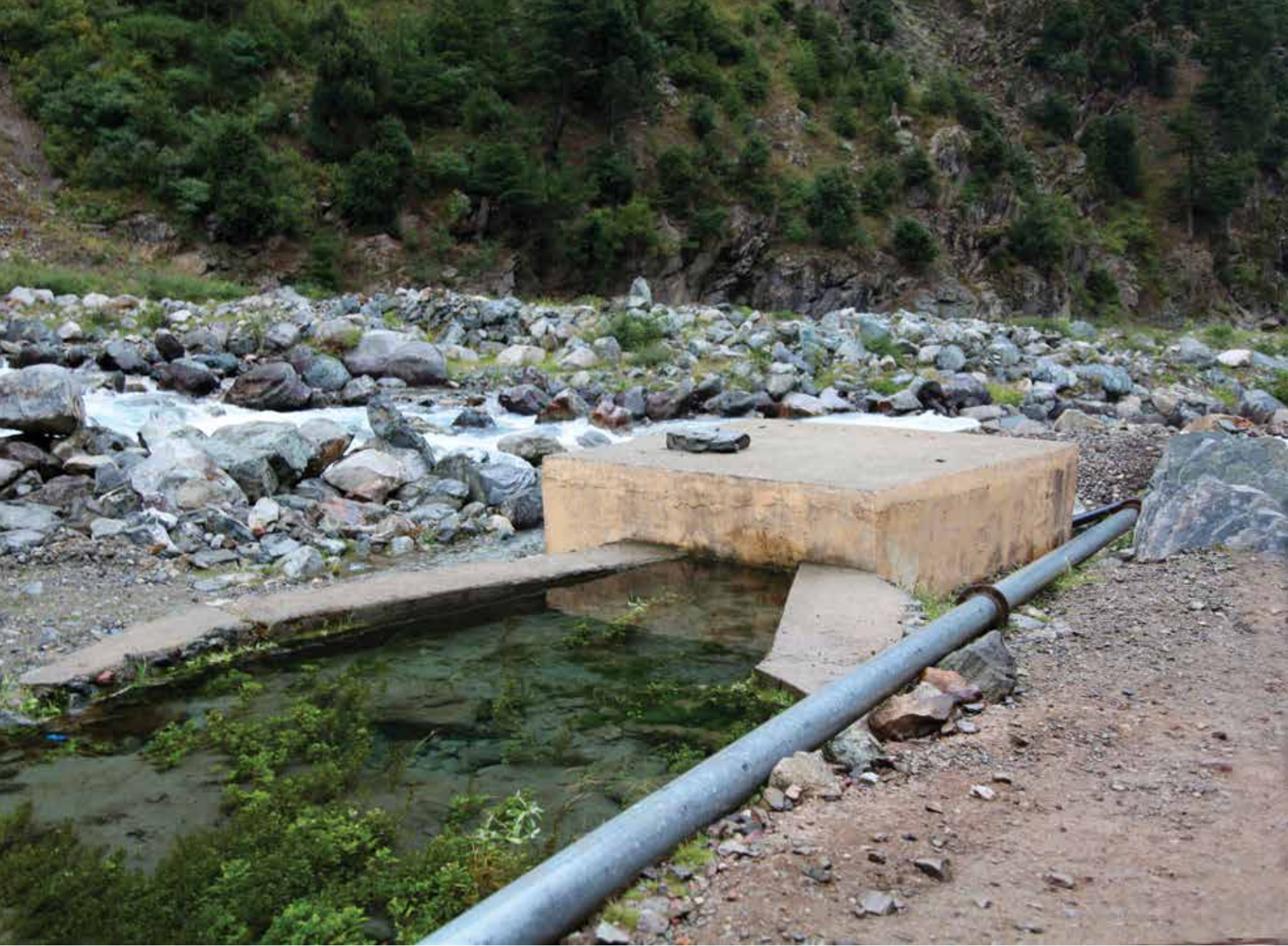
The intake of drinking water with an iron pipe in Anakar valley for supply to the Kalam village. 2019.
