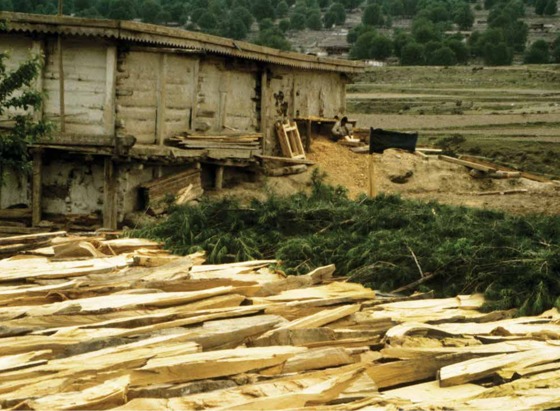
Making a flat house roof with wood put on beam and covered with pieces of brushwood and finally a layer of soil. 1982.
