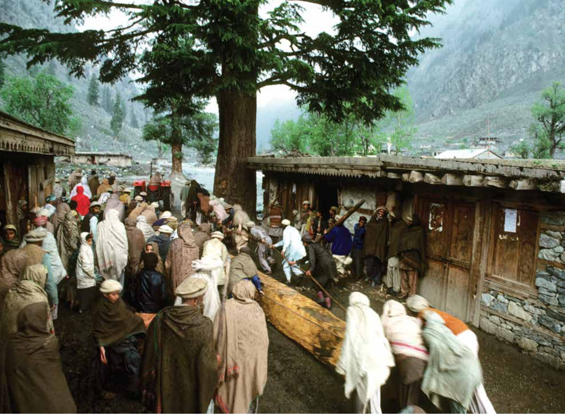
The residents of Bella collectively transport a beam for the construction of a bridge. 1983.
