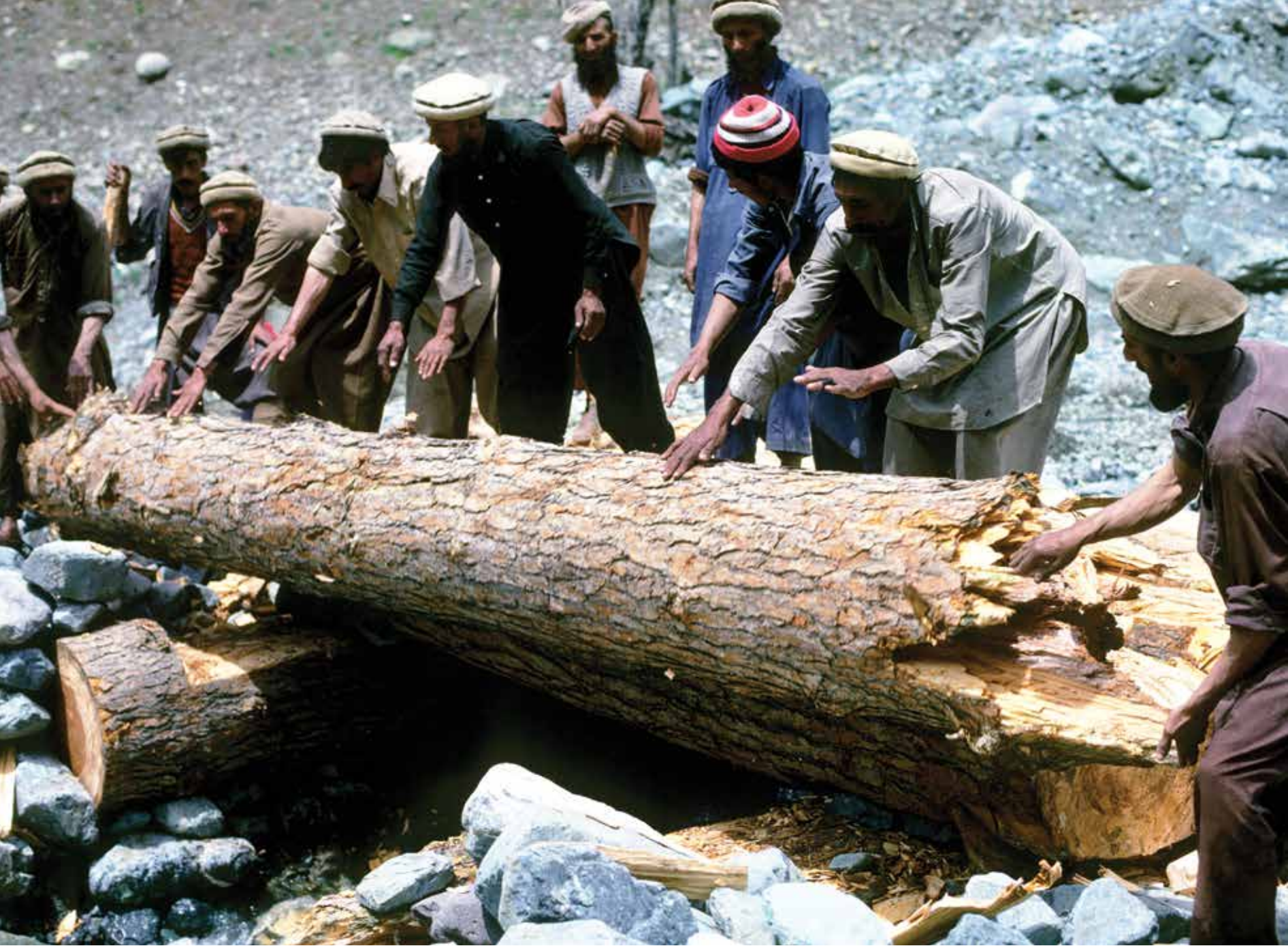
Batandar men repair a bridge damaged by the floods with a tree trunk. 1986.
