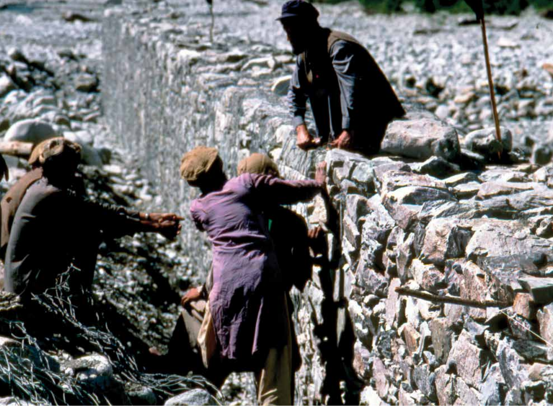
A river protection wall built by KIDP in Anakar valley. 1986.
