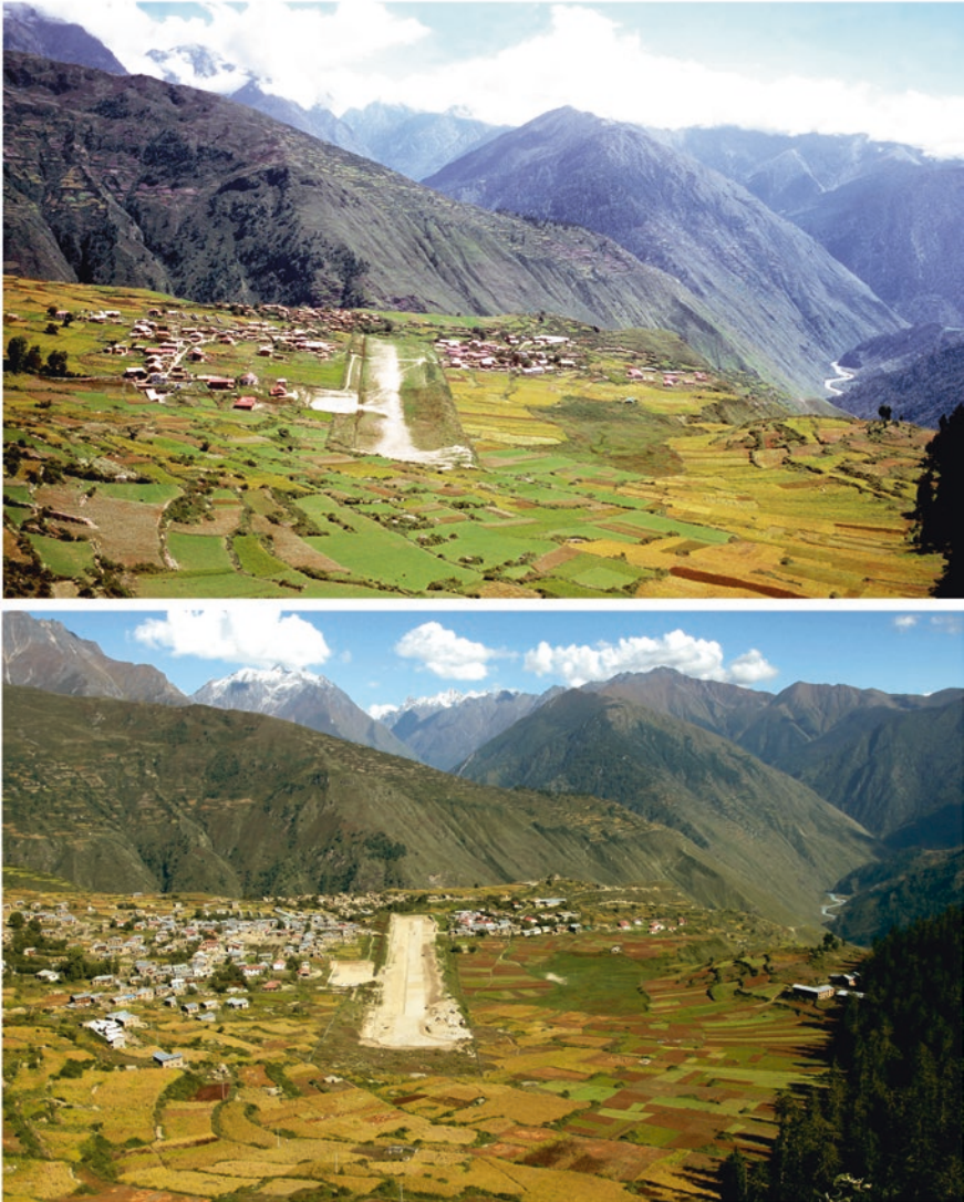
Photo 9.8b The airfield expansion of Simikot, Humla, in Nepal 1999 and 2010 The photo of 1999 shows the narrow unpaved runway. It is surrounded by new buildings in a fertile plateau. At the end of the runway, the old village of Simikot is visible 2010 shows a now-paved runway under construction. Simikot has greatly increased on both sides of the runway. The place now has electricity, which is visible through the line that leads across the fields
