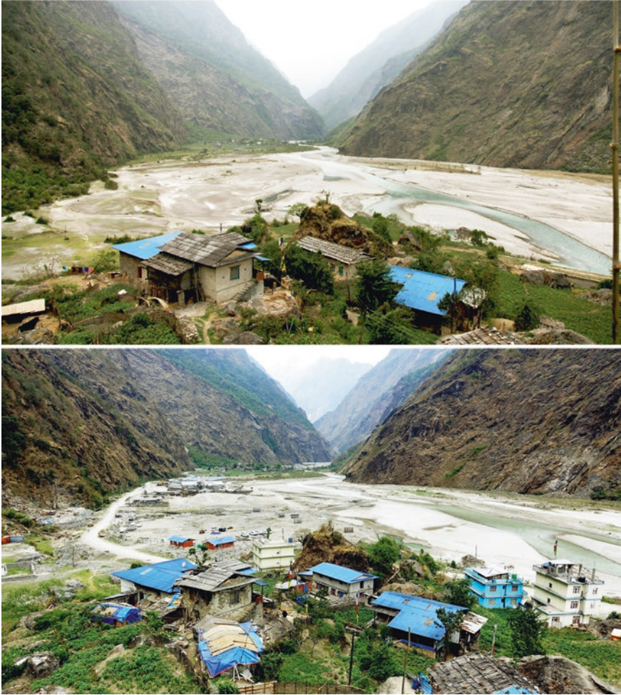
Photo 9.8a A dam is being built at Lamabagar, Nepal 2010 and 2016
