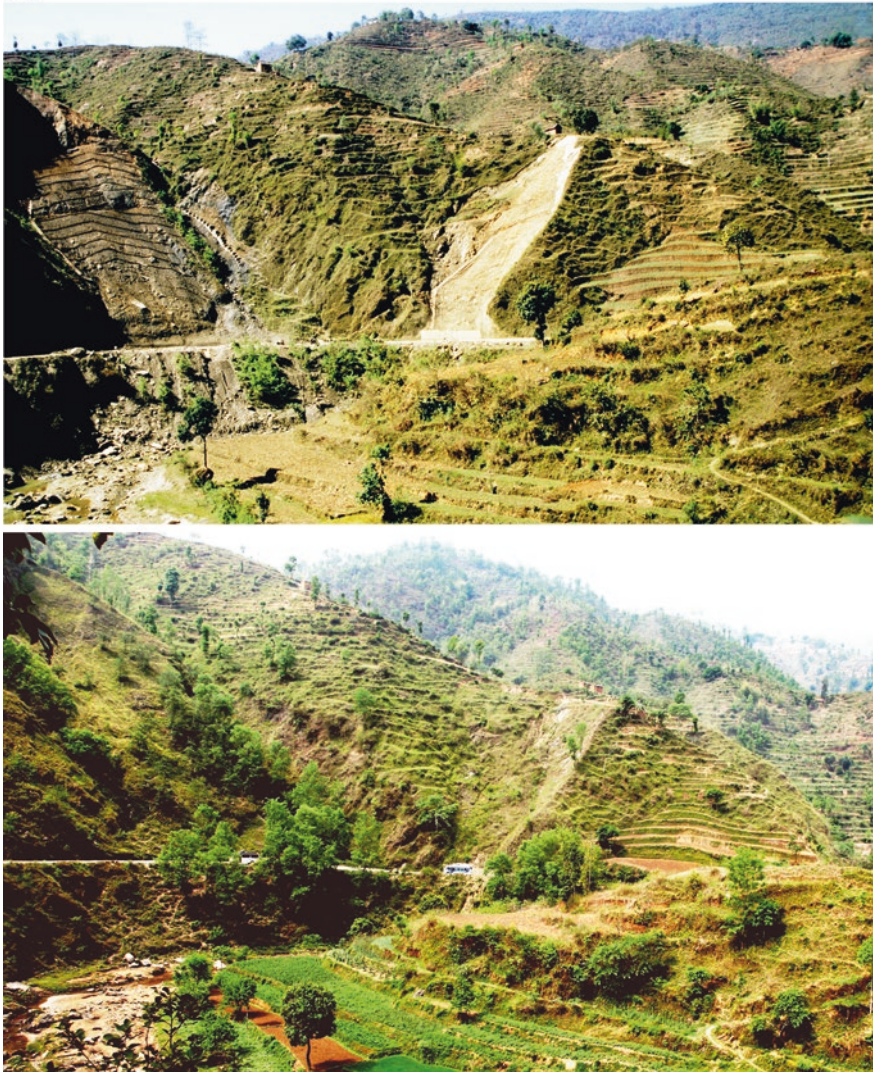
Photo 9.4b Tree planting after the old road-widening construction, Dolalgath, Nepal, 1998 and 2010
